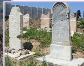
↑ Year 2012: Part of Matzeivos repaired
